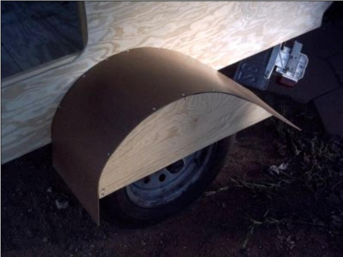
The photo above shows the fender constructed, and the excess waiting to be trimmed. One way to trim the hardboard is the same method for trimming the overhang of the skin material. Take a jig saw and cut the majority of the excess material away. Next use a hand plane to take the hardboard down, and clean up with the belt sander.
