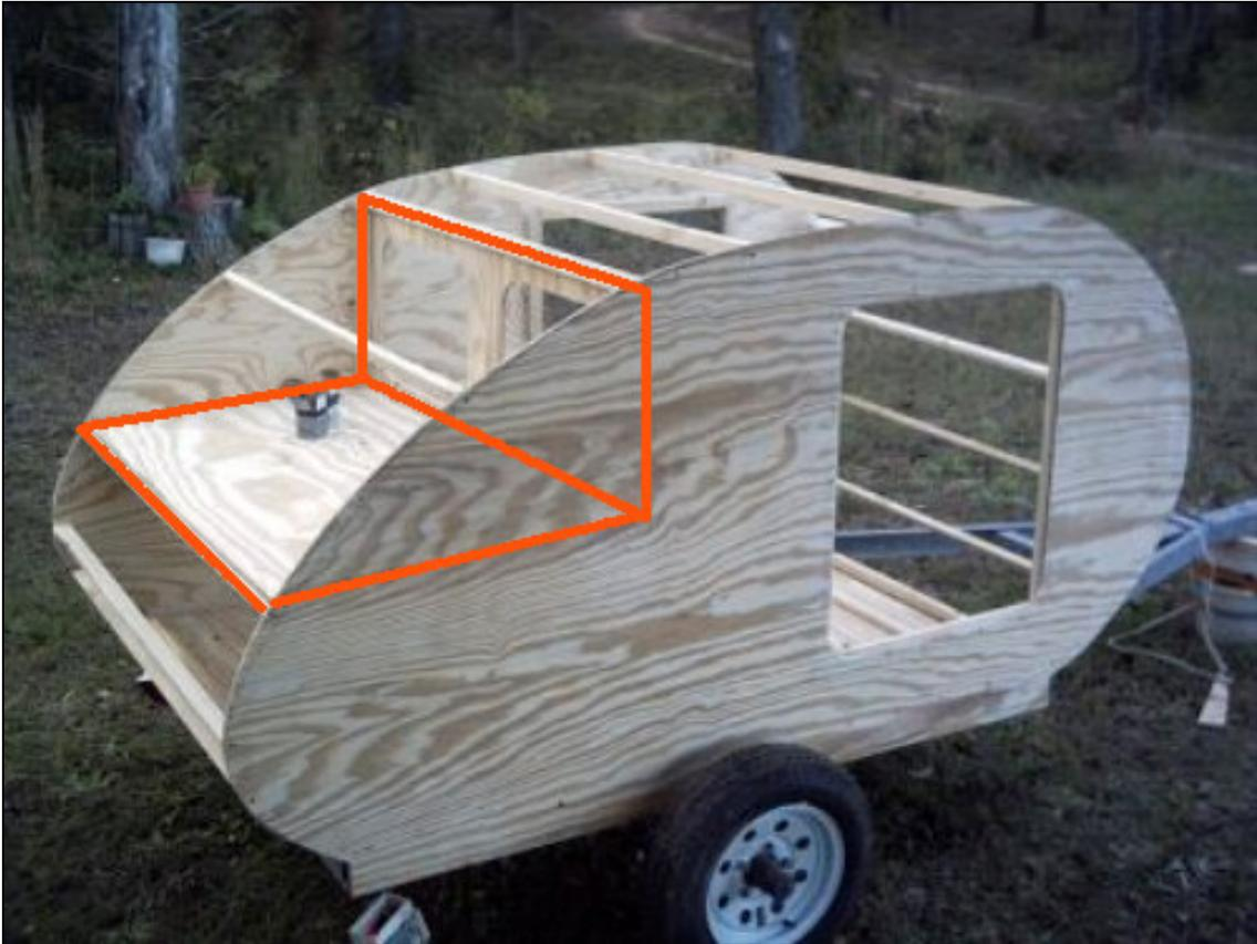
The cupboard is constructed from the leftover  $\frac{1}{2}$ " plywood that was used in constructing the floor.
